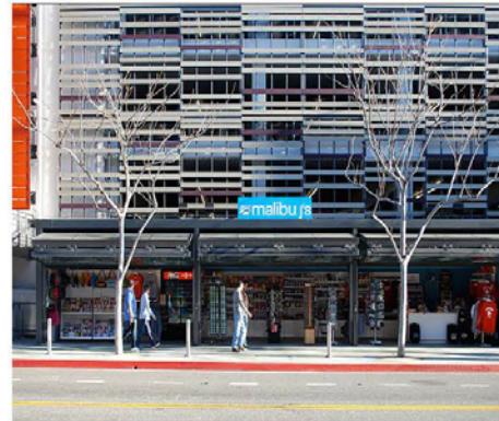
Figure 7 This garage uses architectural elements to screen cars at the upper floors while providing retail at the ground floor. Photo Credit John Edward Linden.
